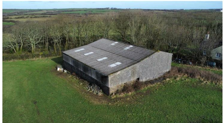
This is situated a short distance from the Bungalow and comprises a steel portal frame within infill block elevations to part with corrugated cement fiber clad elevations and roof. There is a roller shutter door together with a personal door providing access to the side and with a further door to the fore and part of the floor as been concreted whilst the other area is compacted stone. This building provides useful storage for machinery or livestock.
